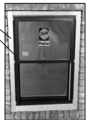
Photo C Brick veneer application
